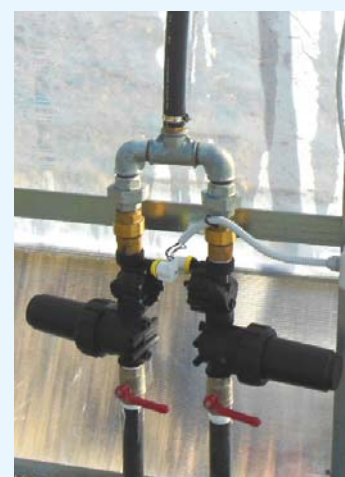
Double water-feeding group , ball valve, net filter and solenoid valve.
